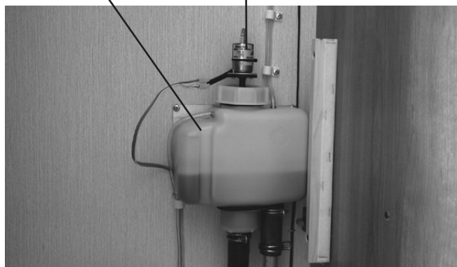
Expansionskärlet Cirkulationspump
