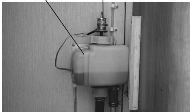
Expansionskärlet Cirkulationspump
