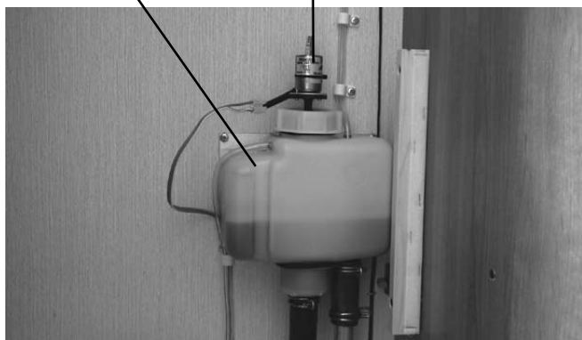
Expansionskärlet Cirkulationspump
