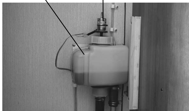
Expansionskärlet Cirkulationspump
