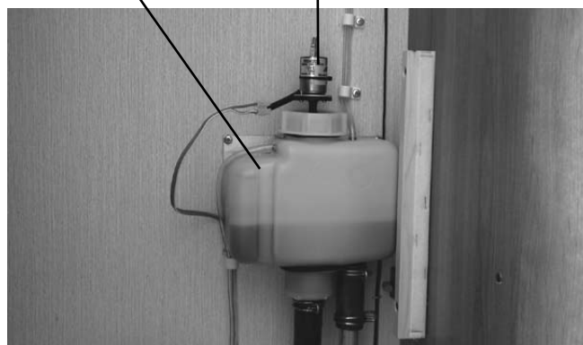
Expansionskärlet Cirkulationspump
