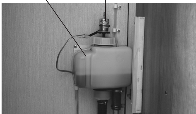
Expansionskärlet Cirkulationspump
